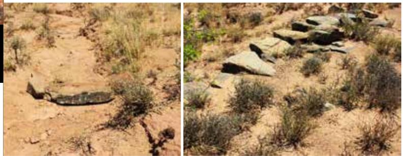
**On the left, one can see flat stones packed inside a water eroded gully to slow down the water flow during the next rainstorm. On the right, one can see how the silt has built up behind the layers of stones**
